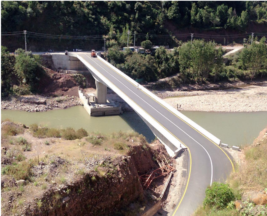
BALANCED CANTILEVER BOX GIRDER BRIDGE LANGARPURA AJK
