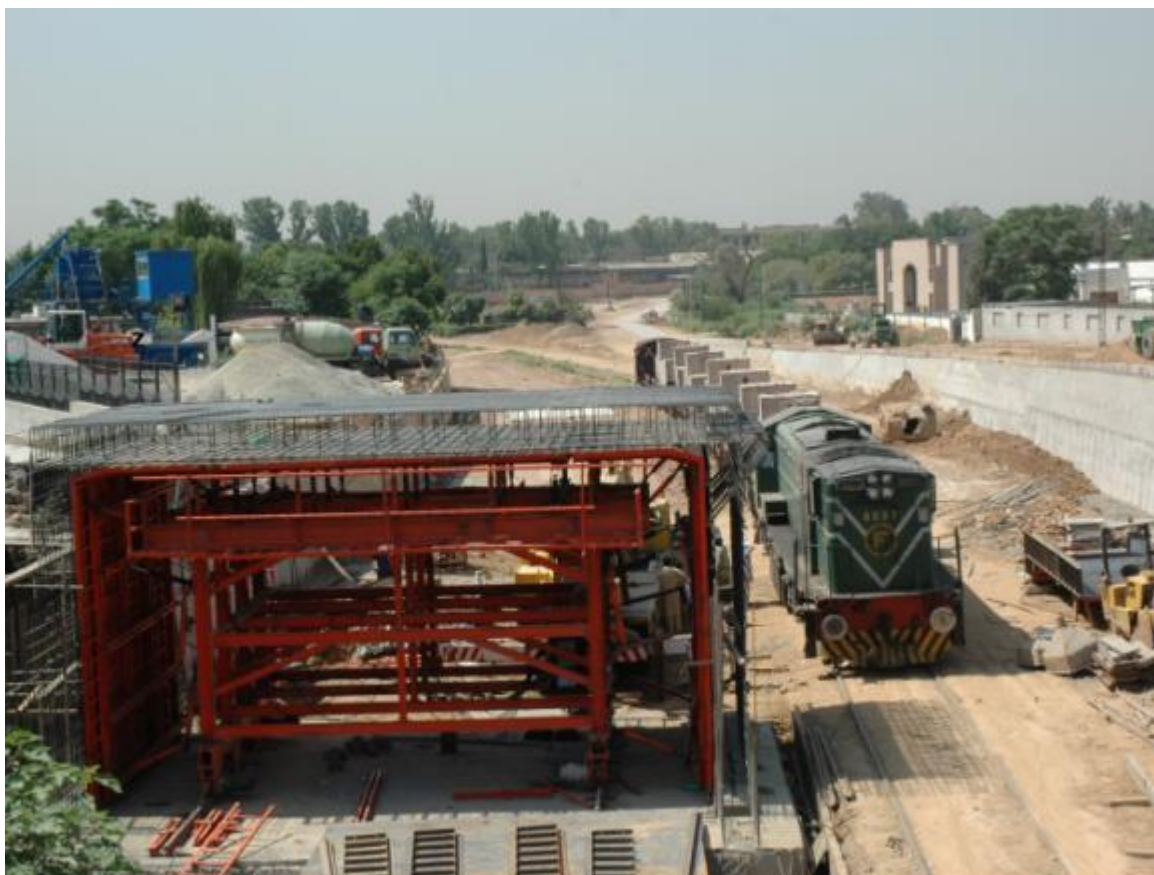
TUNNEL FORMWORK FOR THREE CELL BOX CULVERT AT JUNCTION OF ADYALA ROAD AND N-5, RAWALPINDI
