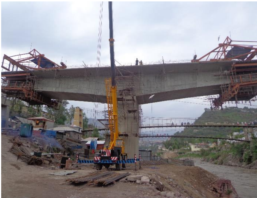
BALANCED CANTILEVER BOX GIRDER BRIDGE JALALABAD, AJK
