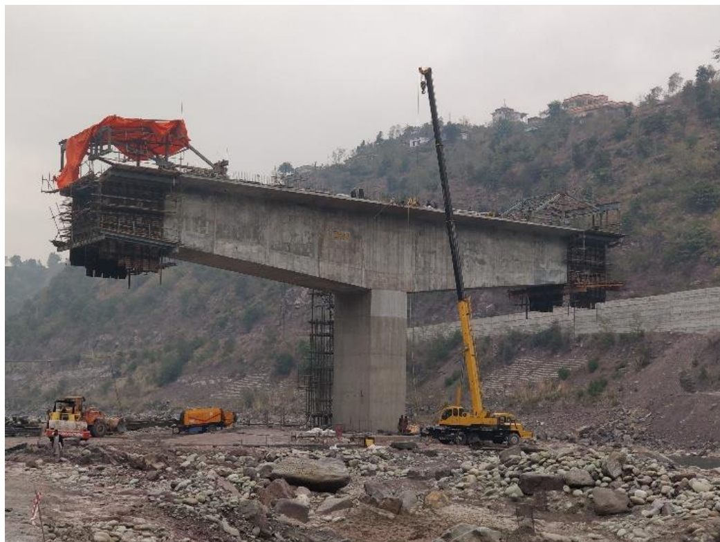
BALANCED CANTILEVER BOX GIRDER BRIDGE KOTLI TATTAPANI ROAD
